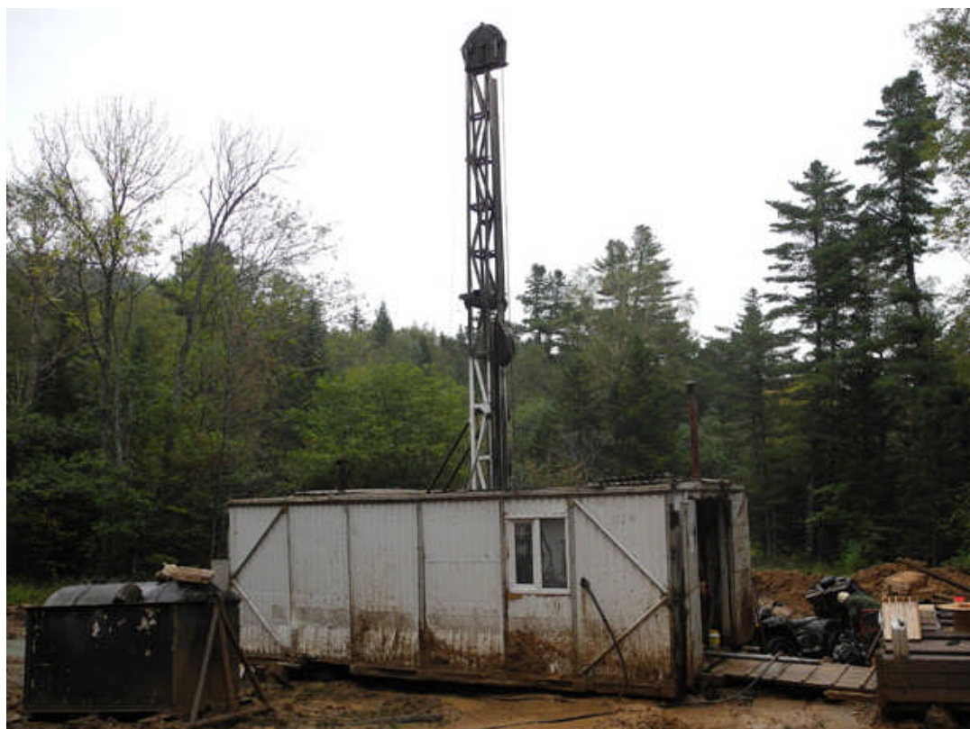
Photo 10.1: LF90 Drill Rig at the Valley Deposit
